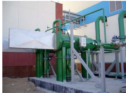
24" / DN 600 KAF Filter seawater cooling
